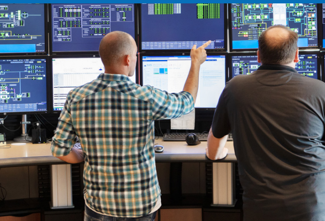
Controllers at our Operational Control Centre
