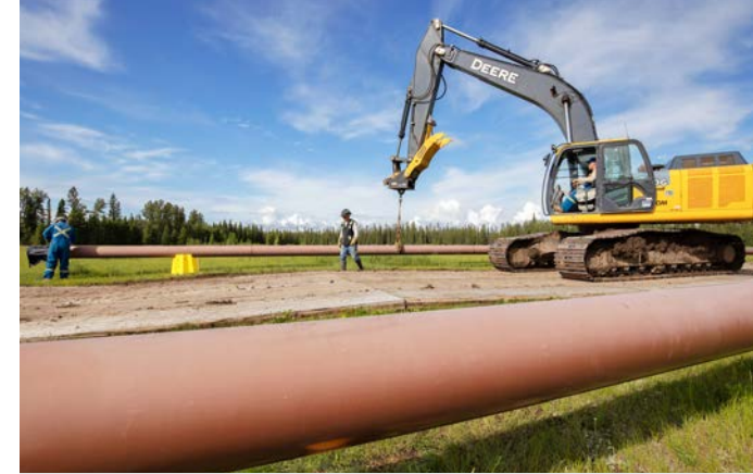
PMC crews preparing pipe for HDD
